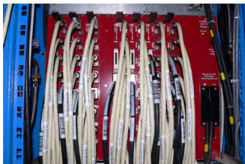
Figure 2. Installed RCT Crate.
