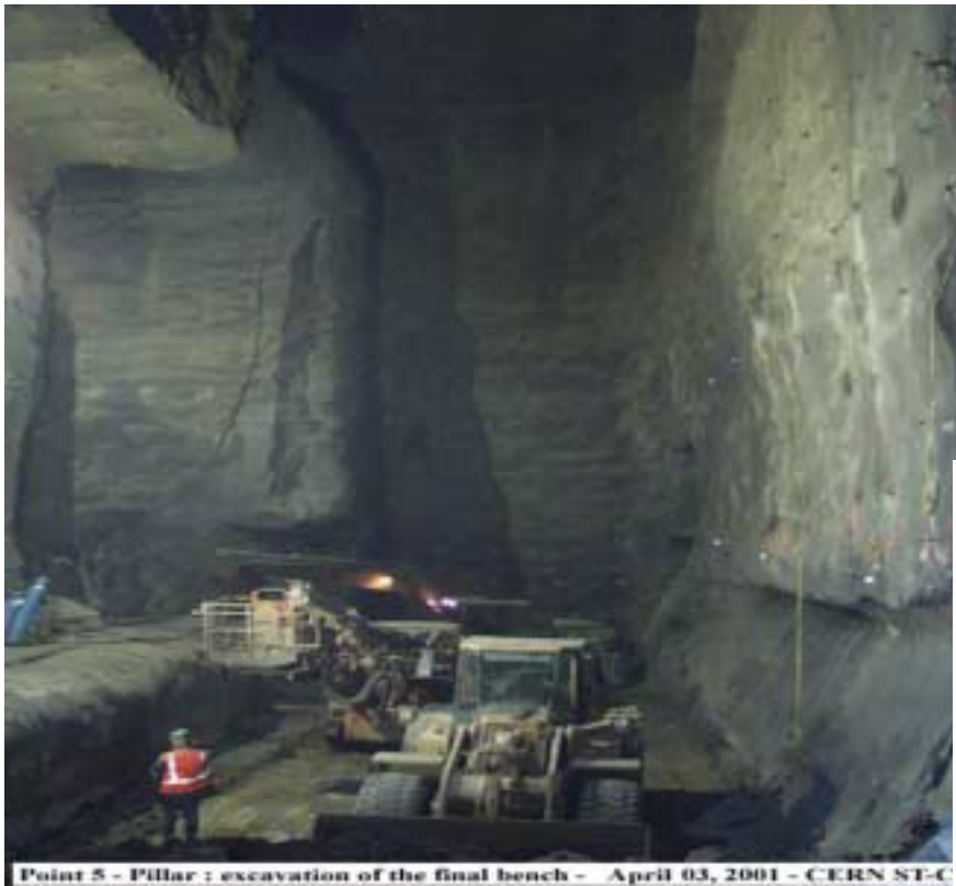
Point 5 - Pillar : excavation of the final bench - April 03, 2001 - CERN ST-C
