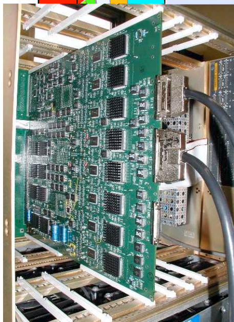
Crate Rear: Loopback Cables to test inter- crate data sharing
