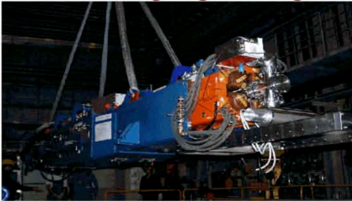
A final focusing magnet being installed
